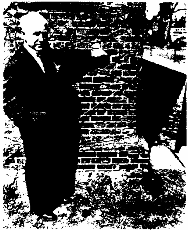
FIG. 2. Stanley Newman examining original lime mortar at Massachusetts Hall, after 240 years of exposure in severe New England climate.
